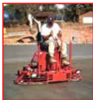
Operator at Work with the Ride-On Trowel
